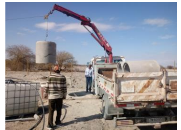
Process of making the well.
