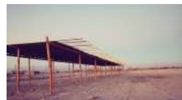
Construction progress at camp.
